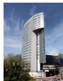
Tech Gate Tower Parkgarage, Wien, Donau City
